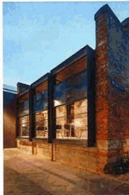
Lit tenancy window displays
