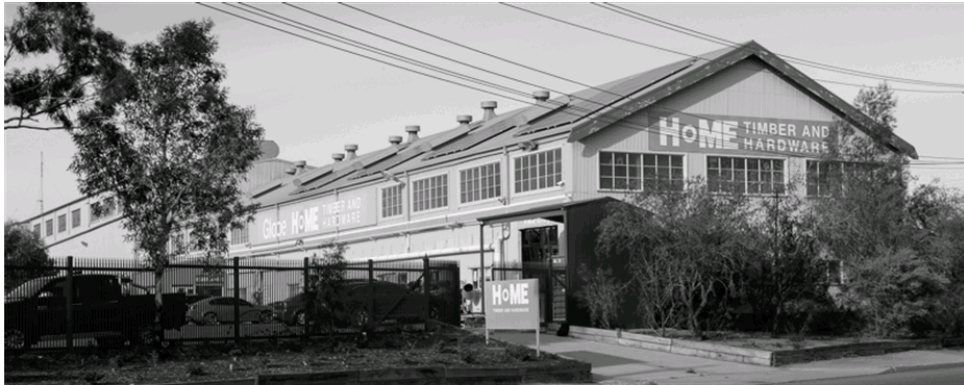
Figure 57 : Former Tramway power station in Galena Street.
