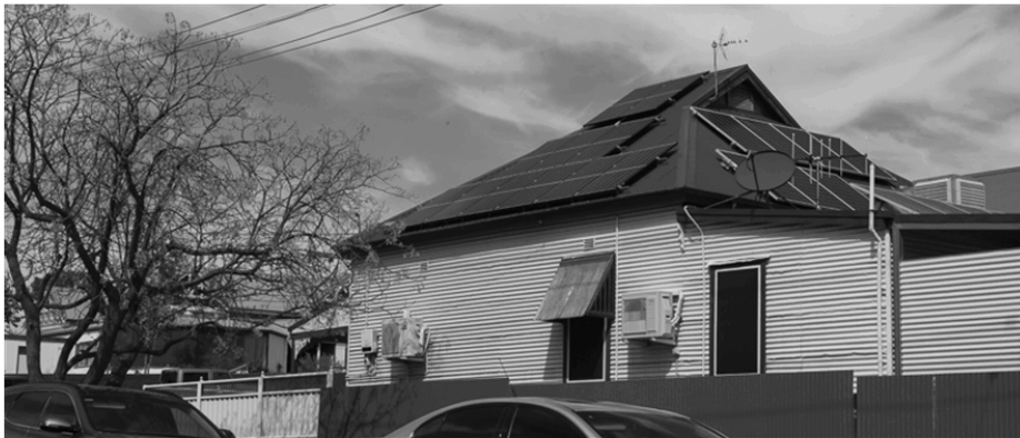
Figure 75 : This example of a solar installation is provided as it illustrates the visual impact of installations where they are highly visible from streets. The site is not a heritage item or within a heritage precinct but is opposite a heritage site. The current Council controls do not require consent for such installations outside heritage sites.
