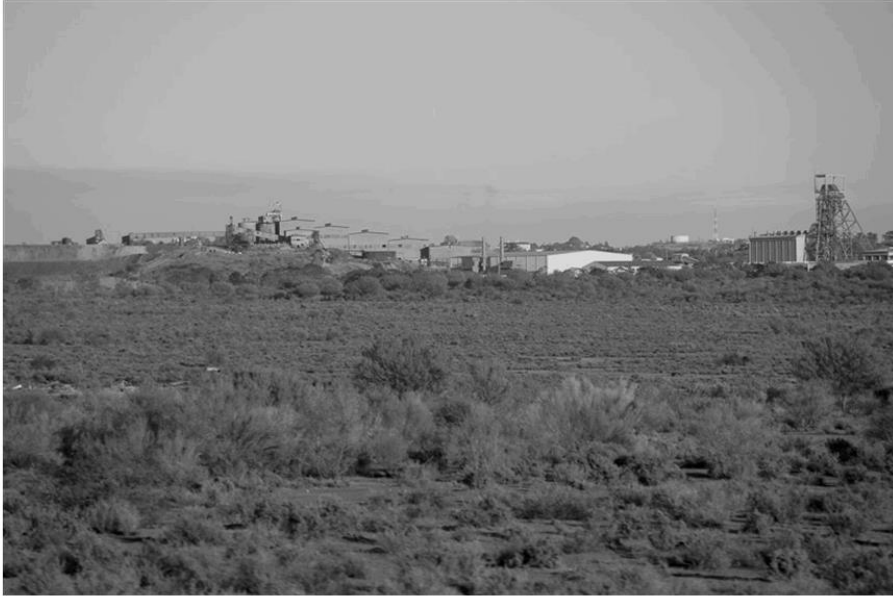
Figure 10 : North Mine with the imposing Mill Building 2 in the centre ground viewed from the north-east on the verge of the Barrier Highway. This view meets visitors as they approach Broken Hill from Sydney.
