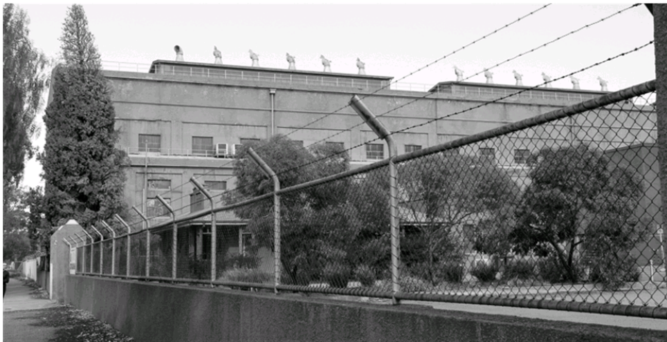
Figure 56 : Former Mine Power station in south Broken Hill, more recently used for film studio use.
