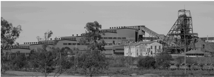
Figure 9 : The north Mine Mill Building and No 2 Headframe viewed from Argent Street where the structures dominate the skyline. Most of this infrastructure is unused and abandoned.
