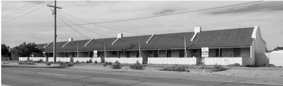
Figure 26 : A row of 6 terrace style houses (forming part of a larger complex in three streets). This form of housing is rare in the City with only a few examples. LEP Heritage Item as a group, noting that the other adjoining examples are not heritage listed.
