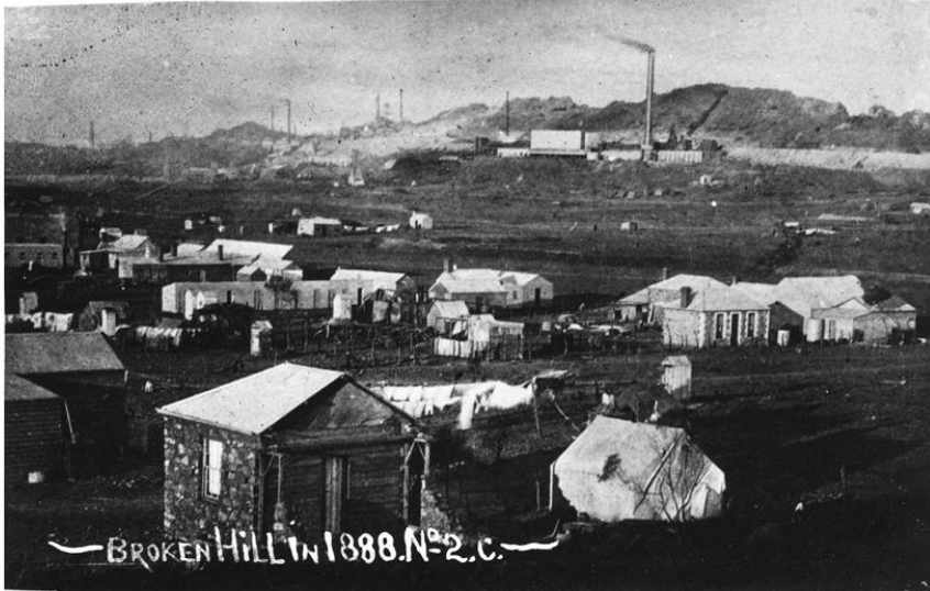
Figure 16 : Dwellings in 1888 showing more detail of the type of buildings being erected. Note in the foreground a tent and a partially complete stone dwelling with a range of stone and timber/iron buildings beyond. Roof forms vary from skillion to hipped to gabled. BH 280
