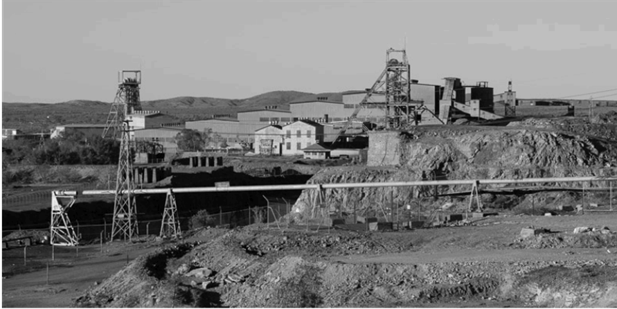
Figure 8 : No 2 Headframe and the Mill Building viewed from Browne's Lookout and shaft looking north-east. No 3 Headframe is in the background. Other elements also appear in the photograph. Taken from a popular lookout, where there is interpretation of the view available, the remaining structures provide an impressive mining landscape that contains the last of the major mining buildings and features. The Mill Building dominates the landscape from all directions as illustrated below.
