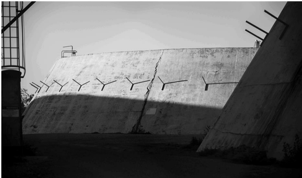
Figure 45 : Early concrete water tank above Block 10 mine site.
