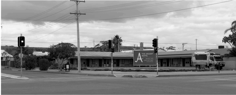
Figure 39 : Criterion Hotel (called Argent Motel on the sign) site showing the retained motel wing to the rear and the now vacant corner.
