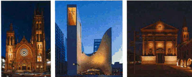
Spotlights mounted to smart poles to light onto select heritage façades. Luminaire selection have narrow beam/ asymmetric lens optics to highlight key features of buildings.
