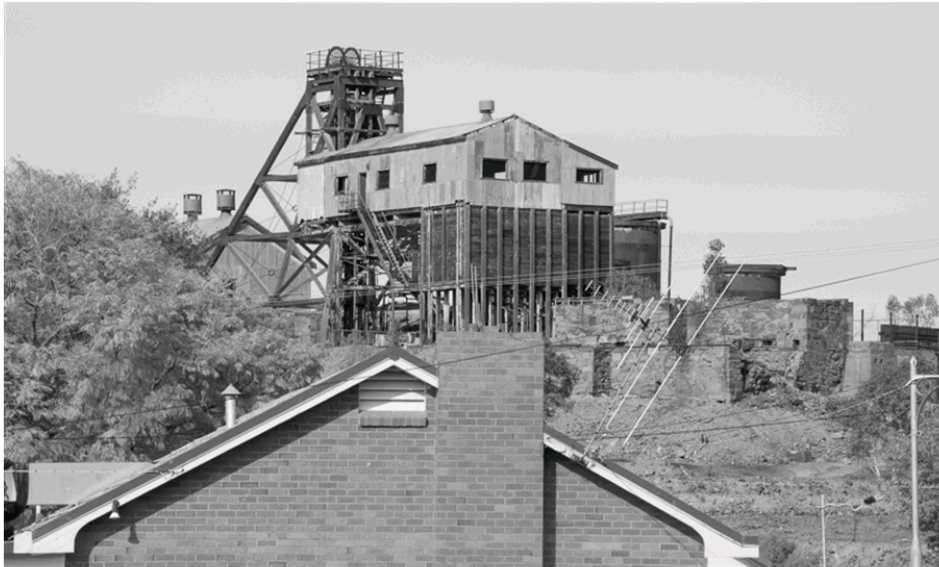
Figure 7 : Brown's Shaft/Junction Mine above Junction Circle housing. The mine is abandoned and a public lookout with interpretation. It is presently in fair condition but the nature of the buildings and elements will result in long-term deterioration and potential loss unless there is ongoing, consistent and significant investment in the site.
