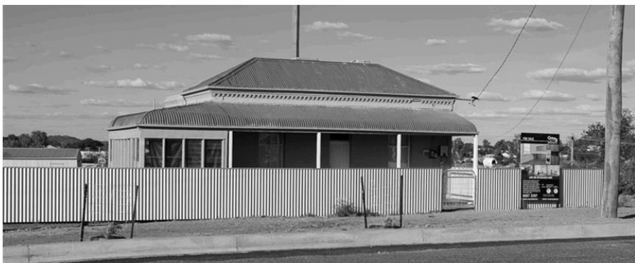
Figure 28 : A modest but well-detailed house with return verandah in North Broken Hill. The building is not heritage listed nor within a heritage precinct.
