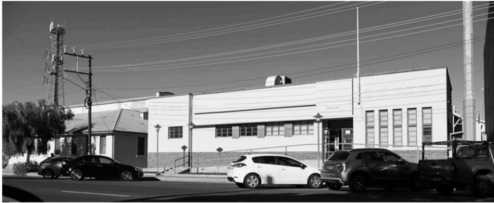
Figure 44 : Water Board Building in Blende Street
