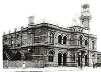
Broken Hill Town Hall Prior Demolition in 1972
