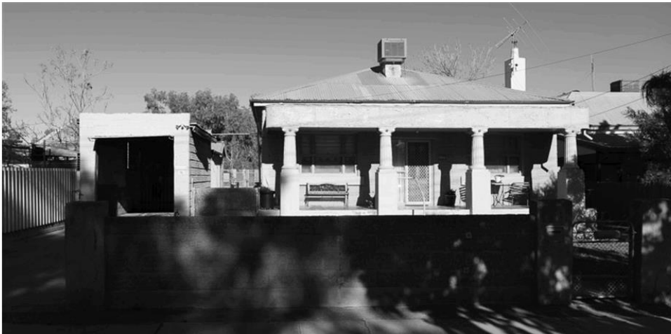
Figure 23 : A typical early timber residence with a later 'grand' verandah added. It is not heritage listed nor within a heritage precinct.
