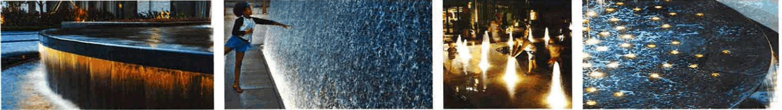
Water feature lighting
