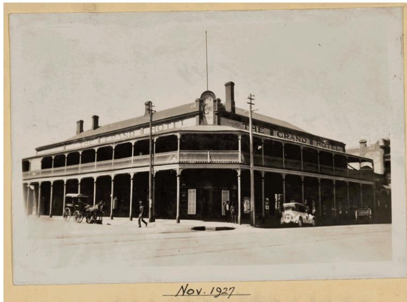
Figure 36 : Grand Hotel 1927 in Argent Street. It has had its verandahs removed with façade alterations since this photo was taken. Noel Butlin Archives, ANU.
