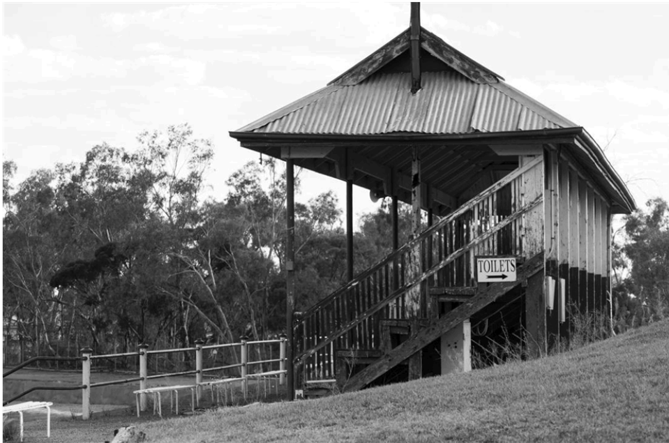
Figure 58 : Grandstand at Zinc Oval, a bespoke structure built on a mining lease by a mining company. Note the seats and railings also built from mine material.
