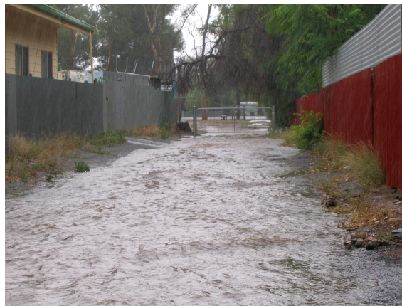
Photo 4 Looking downstream from Patton St along the open channel
