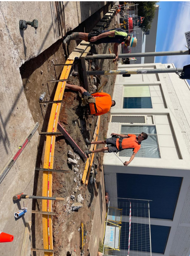
Photograph: Site works commenced – 13 May 2024
