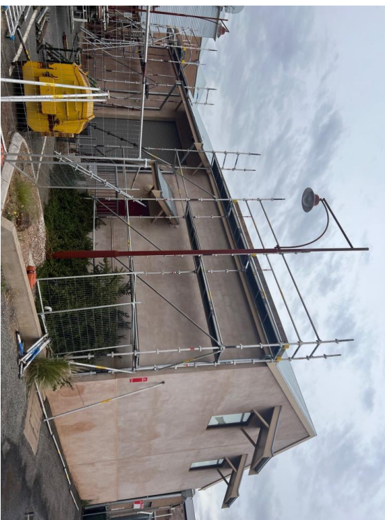
Image: Art Gallery Roof Replacement November 2023.
