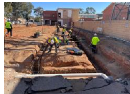
Image right: Steel fixers working on preparing footings
