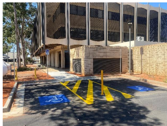
Image above: New accessible parking within Council car park
