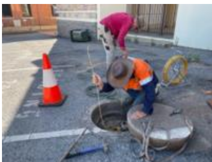
Image left: Site establishment works with services location underway
